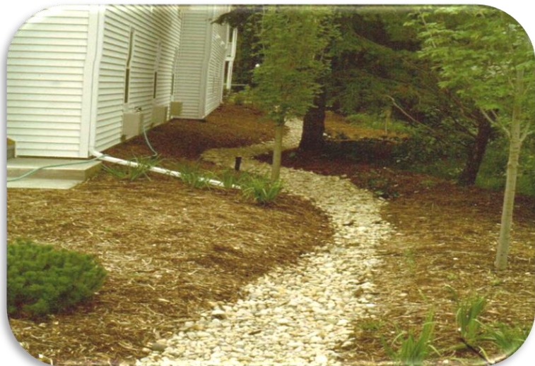
Infiltration trench to recharge roof runoff.
