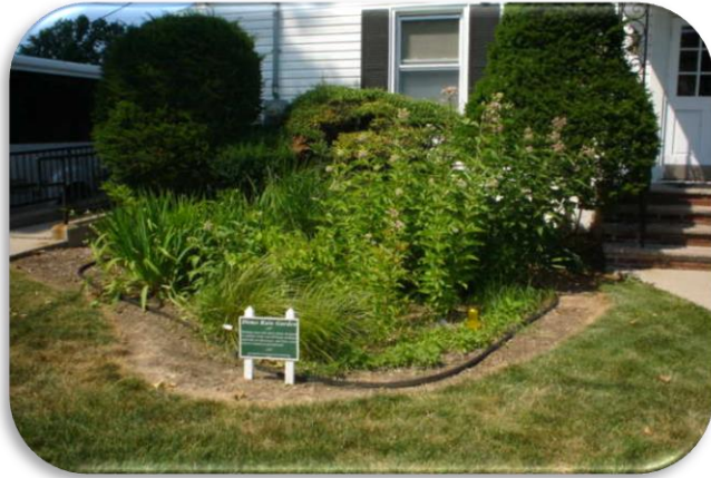
Rain garden installed in a residential setting to capture driveway and roof runoff.
